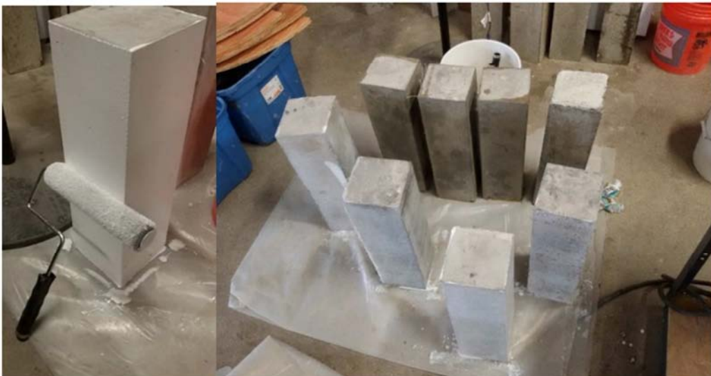
Figure 1. Pictures of a Fiber Reinforced Concrete Beam after the Application of Liquid Polymer Coating.
